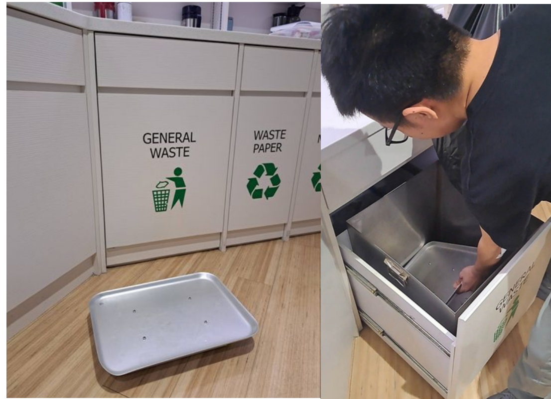
Deployment of bin monitoring system at Grade A office building
